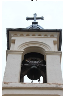
Bell tower detail
